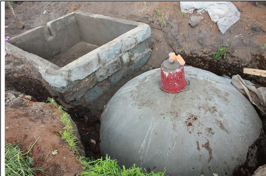
Figure 1: Fixed-dome biogas digester built into the ground
